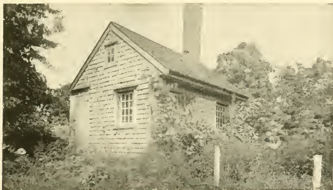
JOEL WILLCUTT'S COBBLING SHOP, ELM STREET. Built 1791. Used as post office 1806 to 1837.
